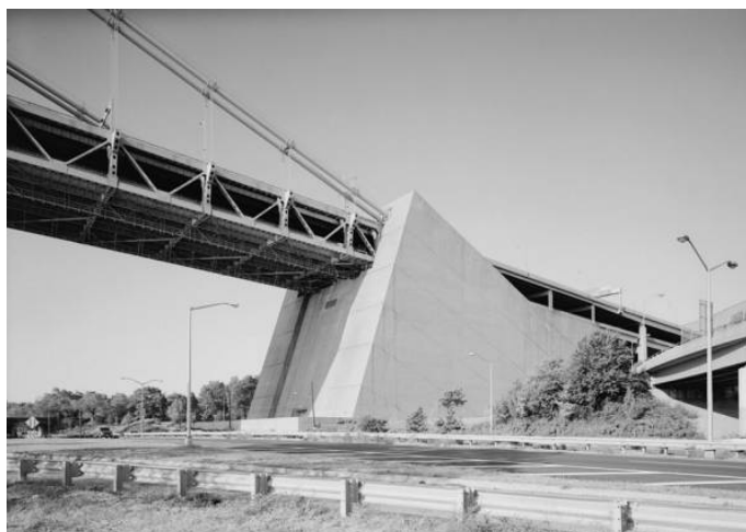
Crtež 4.36: Sidreni blok Mosta Verazzano narrows, SAD
